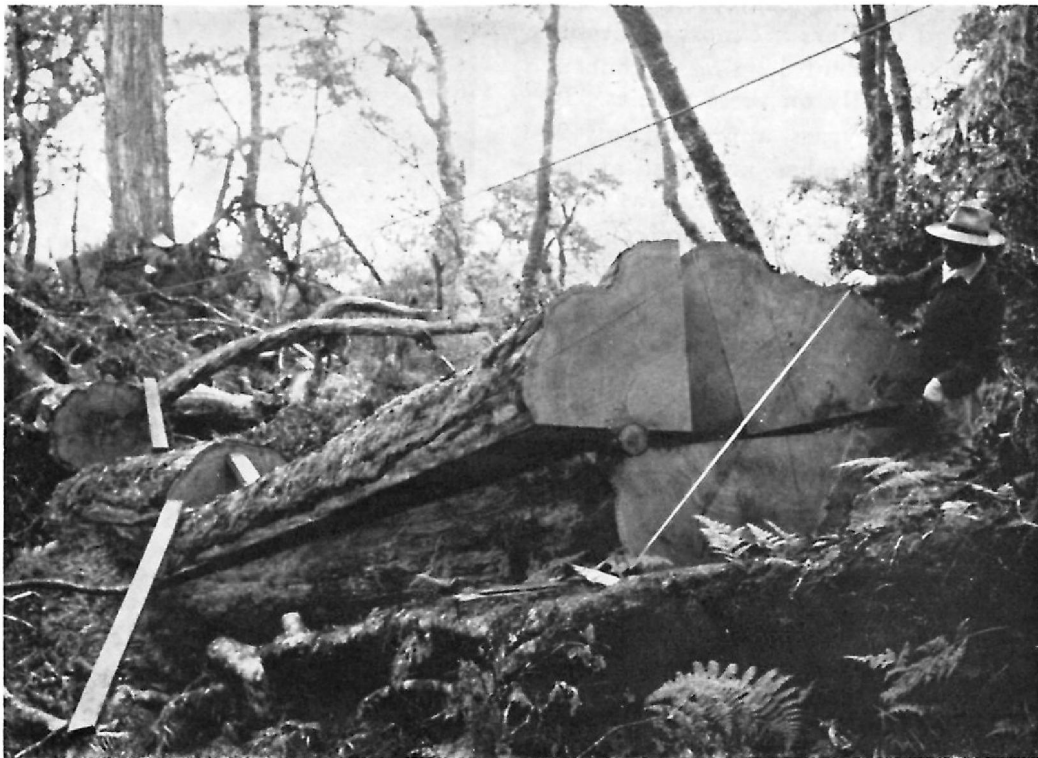
The large logs are ripped in the woods to fit transportation facilities.
