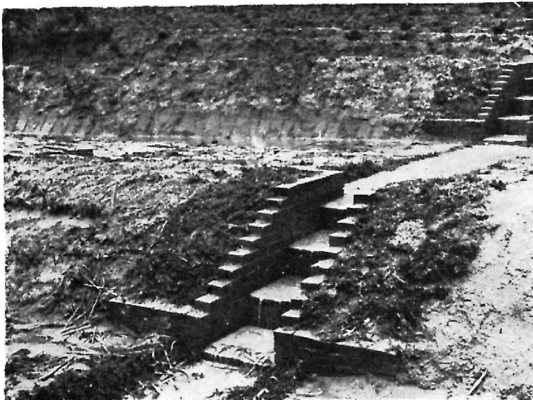
Drop structures made to control the run-off water.
