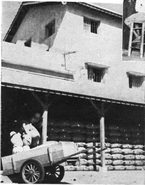
A reinforced concrete warehouse
