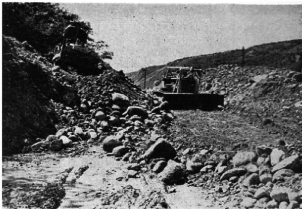
Repair of highway damaged by typhoon
