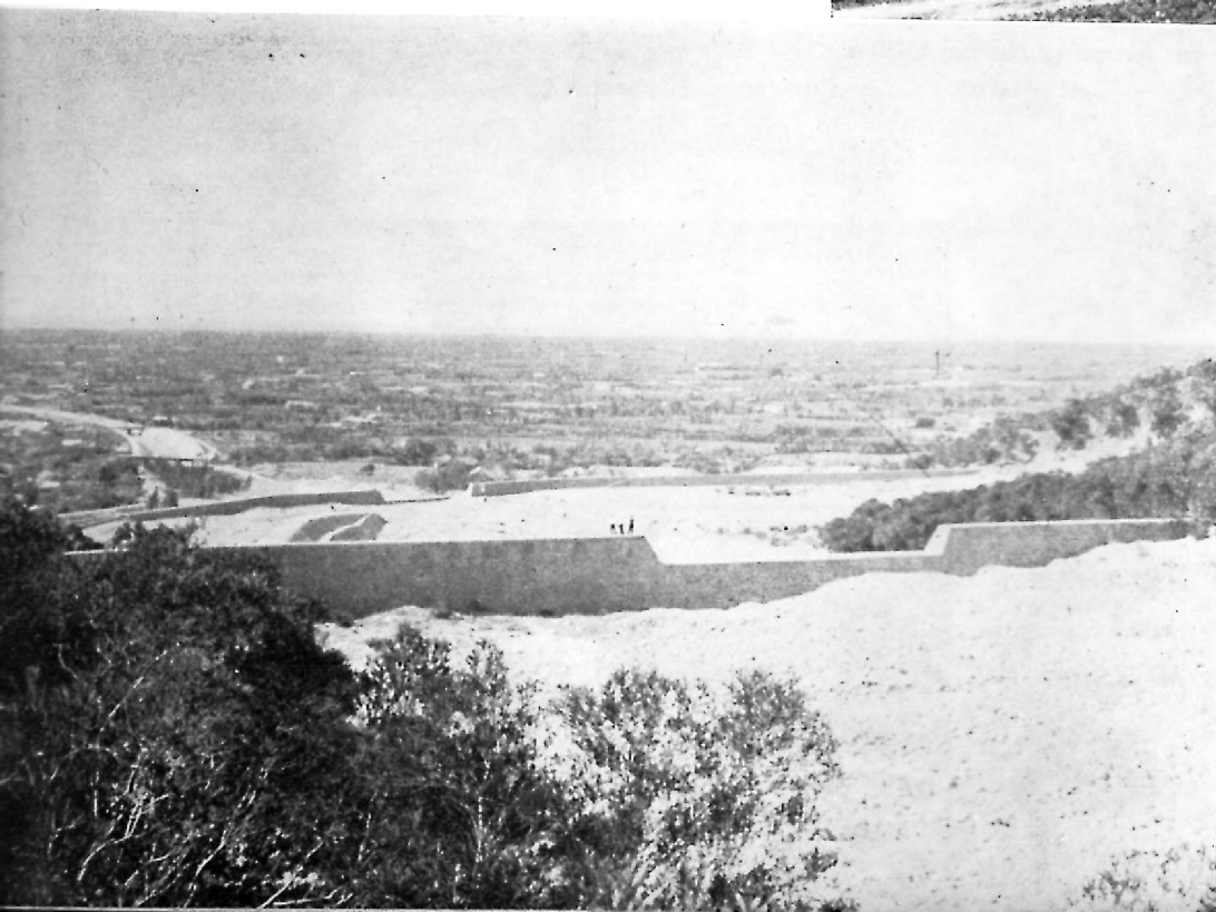
Debris dams such as these provide only a stopgap measure in attempting to arrest sediment movement.
