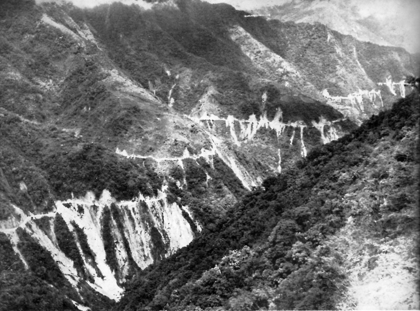
The cross-island highway in central Taiwan caused large areas of exposed soils which are subject to heavy erosion, slumping, and sliding. During and following heavy rainfall it further contributes to flooding and downstream sedimentation.
