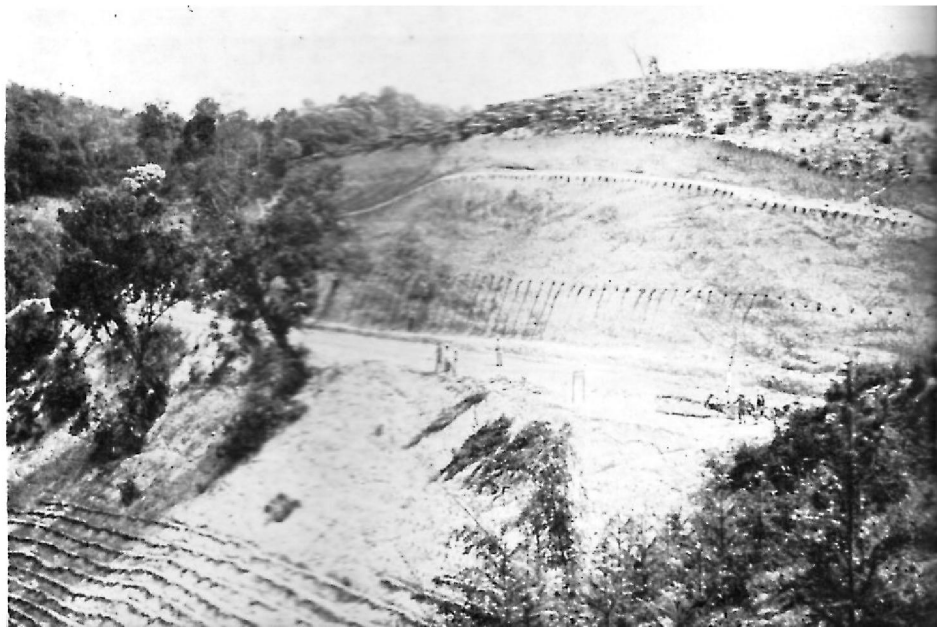
Roads cuts and fills and other areas where sloping soil is exposed should be revegetated immediately following exposure.
