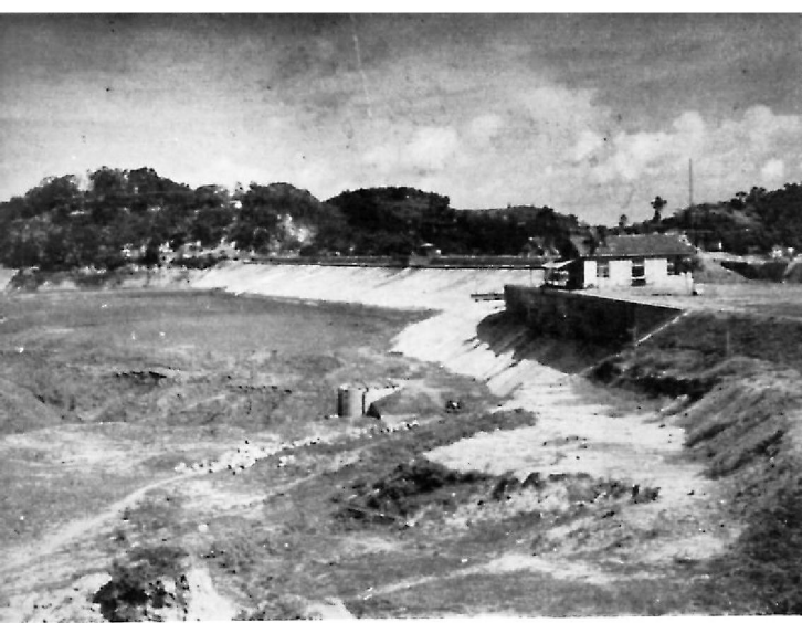
The Gen-shan-pee reservoir, Tainan County, is now soil sediment laden. It has lost much of its value.
