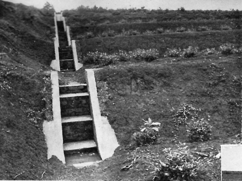
Bench terraces with lined waterway permit the safe cultivation of sloping lands. The risers on this newly benched tea plantation will also be grassed to furnish soil protection.
