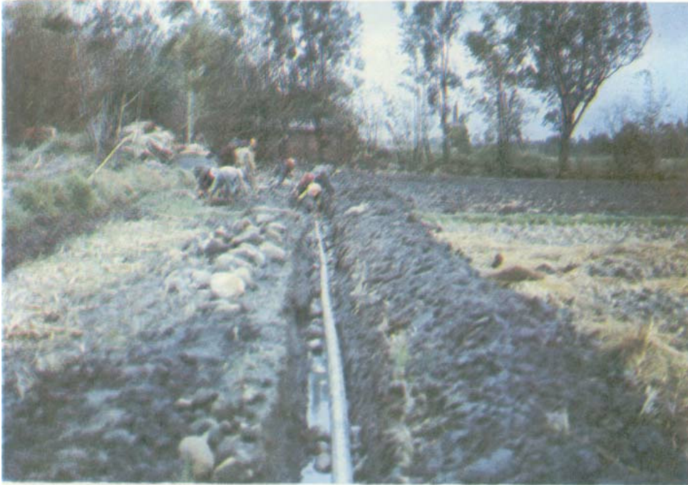
Fig 11: Construction of drainage system is the most effective way for the reclamation of the sandy acid sulfate soils at Ta-an.
