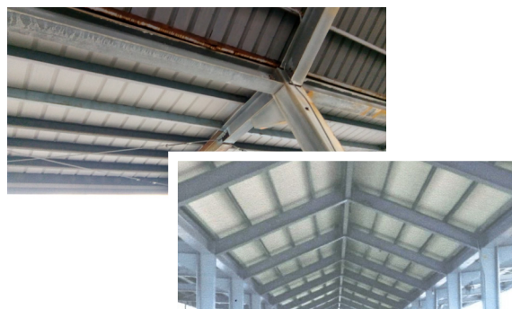
Repair of the leakage from rusting of the gutters, pillars, and beams of the Zhengbin fish offloading site. (Above: before the improvements; below: after the improvements.)
