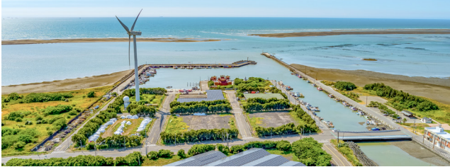
Solar power panels have been installed on the roof of the fishing gear maintenance and repair venue at the Haishan Fishing Port in Hsinchu.
