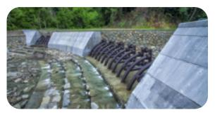
Project to restore a torrent on the Sanchong River: An arch dam with steel tubes, water cascade steps, and an auxiliary dam to dissipate energy and prevent scouring.
