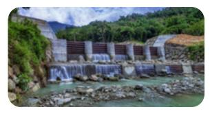
Project to restore a torrent on the Sanchong River: Adjustable check dam and old submerged dam.
