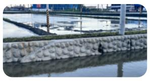
Phase 1 of the improvement project for the Zhuangdong Guting drainage channel includes a ramp for animal life to climb out of the channel alongside its retaining wall as well as ecological tubes, creating an environment friendly to animal life including fish and shrimp.
