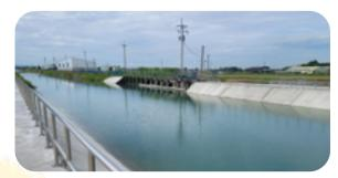
The improvement project for the water culvert for excess water drainage in Nanjing, Chiayi County, used a precast culvert hanging assembly which was built in concert with the lower portion of the Chianan irrigation system. The main construction work on the main channel was completed during a 45-day halt in the flow of water. It helps ensure water transport for agriculture and daily life.
