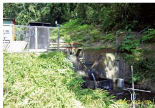
試驗集水區量水堰 An experimental watershed weir.
