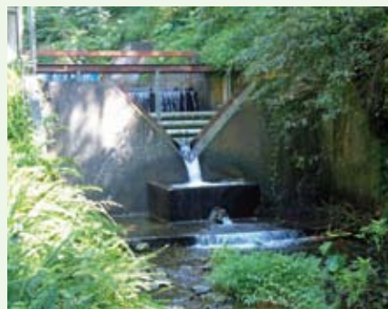
福山1號水文觀測站 No. 1 hydrological station at Fushan.
