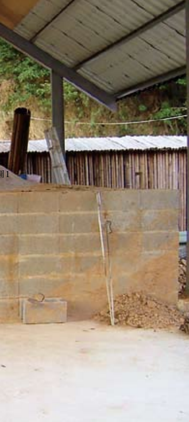
竹炭土窯之外貌與燒製時，每窯所需約250公斤之相思樹薪材 A bamboo charcoal earthen kiln. The kiln needs approximately 250 kg of acacia fuelwood for each firing.
