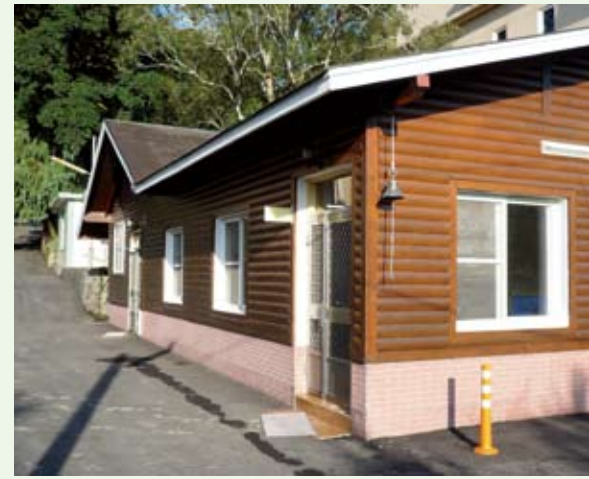
1998年蓮華池研究中心木屋，為框組壁工法與鋼筋水泥混合式構造 Wood building constructed in 1998 at Lienhuachih Research Center, using a hybrid of wood platform construction and reinforced concrete.
