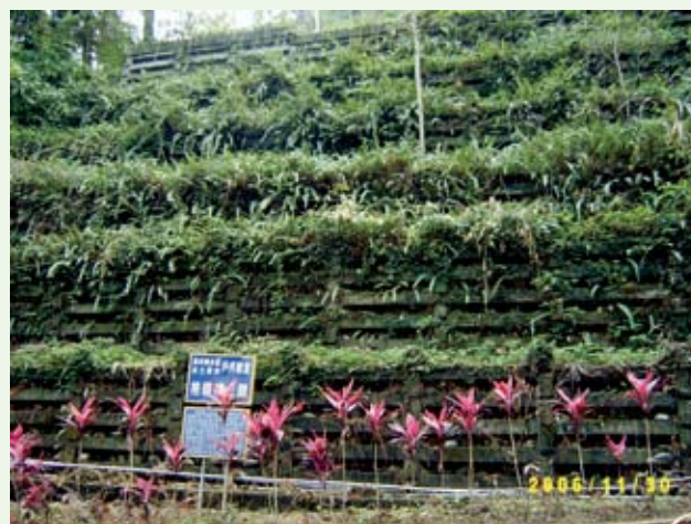
格籠擋土牆 A grid retaining wall.
