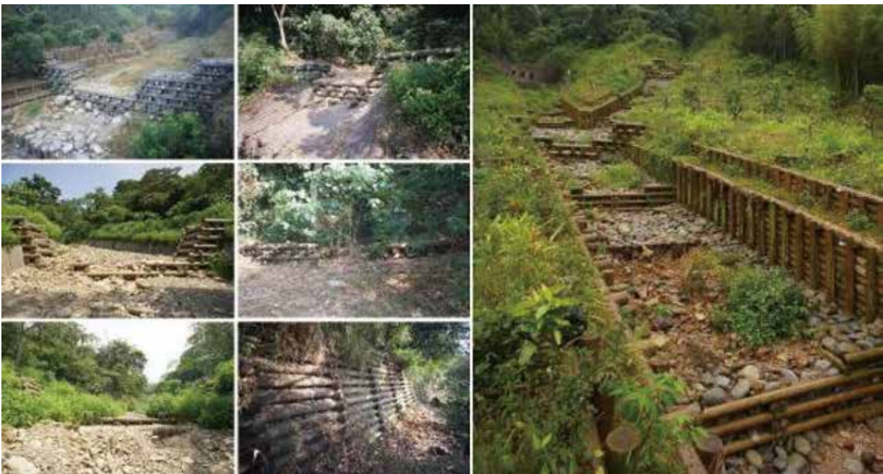
坑內坑與廟前坑森林步道和日月潭所設置之生態工法。 Wood-based material applied in ecological engineering at Nantou.
