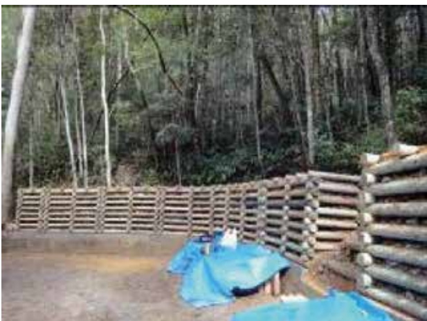
設置護坡牆兩座在蓮華池研究中心(左圖放射松、右圖柳杉) Wood-based material applied in ecological engineering at Yuchih, Nantou.
