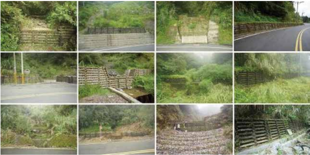
宜專一線沿線所設置之生態工法。 Wood-based material applied in ecological engineering at Yilan.
