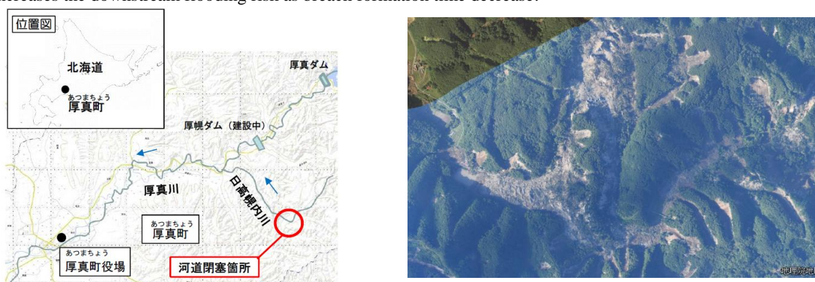
Fig. 1 Location of large-scale landslide at Atsuma Town, Hokkaido, Japan (Geospatial Information Authority of Japan Website).
