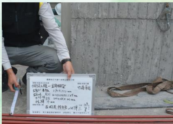
鋼棚架鋼構拉桿施工查驗
