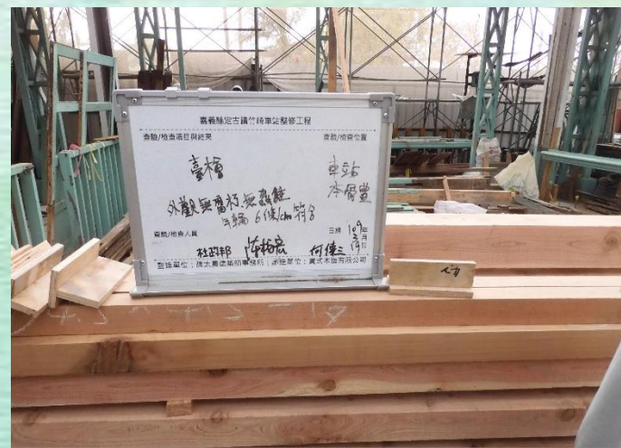
仿作抽換（臺檯）施工查驗
