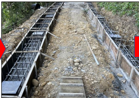
縱樑鋼筋及鐵板銜接
