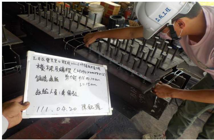
H型鋼剪力釘查驗
