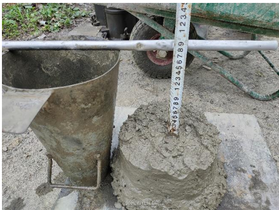
混凝土坍度檢驗
