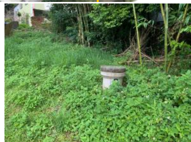
6. 5.1K+250側邊空地抽水井
