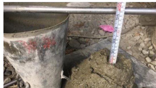
混凝土坍度檢驗
