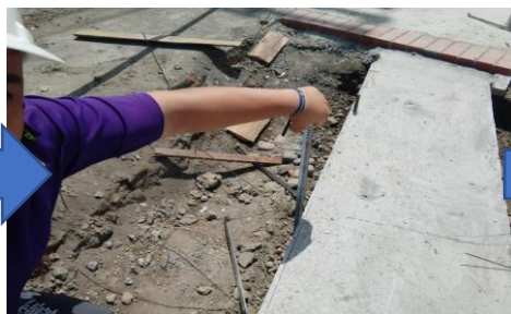
②磚牆基礎查驗
