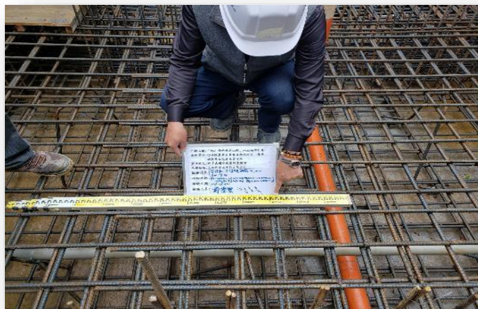
鋼筋施工查驗
