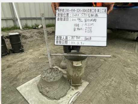
混凝土坍度試驗
