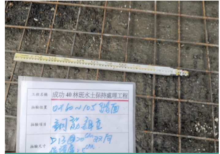
RC路面配筋查驗
