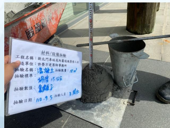
混凝土坍度試驗
