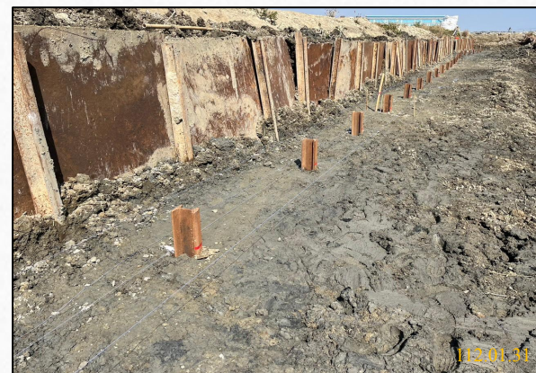
靜壓式鋼軌樁
