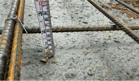
鋼筋主筋#4、副筋#3
