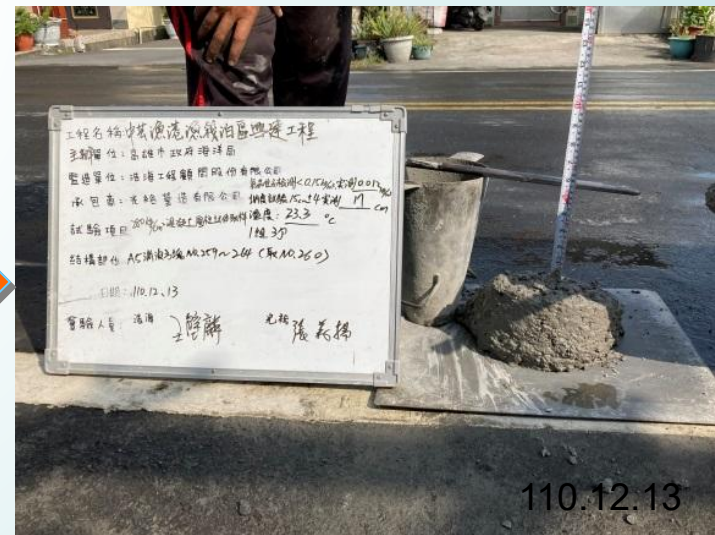
混凝土坍度試驗
