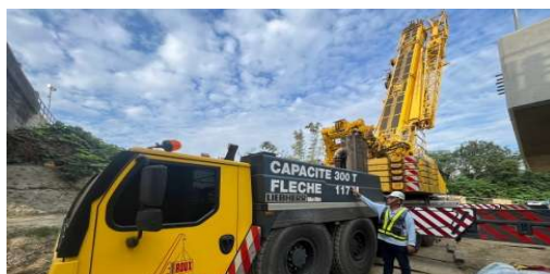
吊車作業前查檢
