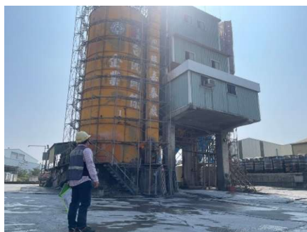
貯存槽設備查驗
