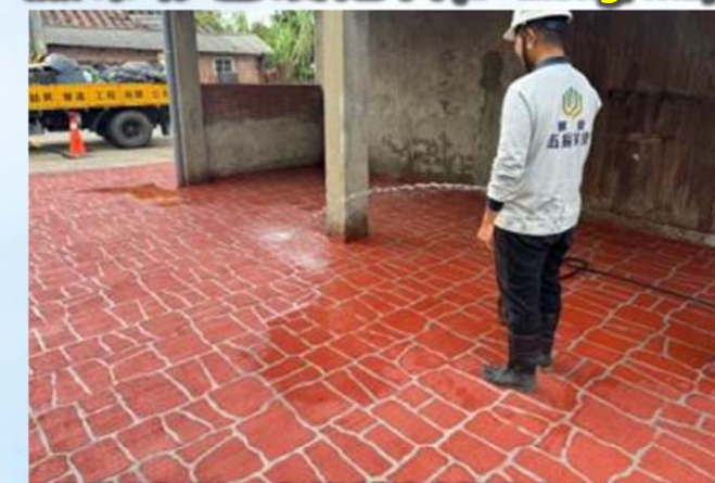
清洗後噴刷養護劑(0.1L/m 2 )
