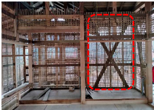
(4)軸組-新作木作牆體筋圍補強
